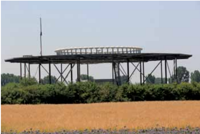
The Doppler VHF omnidirectional range (DVOR) Ried for air navigation services near Pfungstadt (Hesse)
